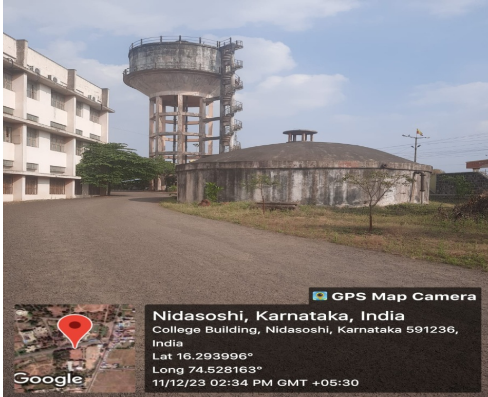
Overhead water tank and ground storage water tank
