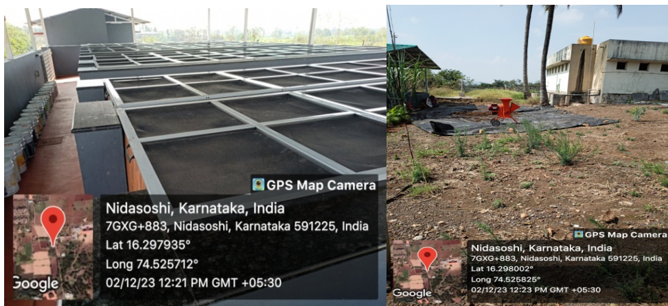
Hermi compost processing chamber Drying and powdering of compost.
