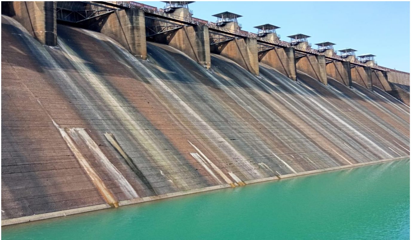
Picture of Ogee spillway
