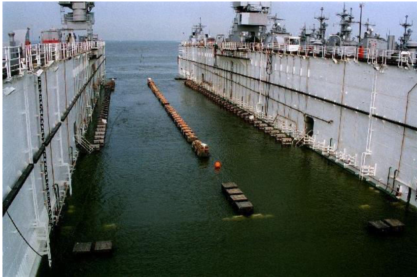
Auxiliary Floating Dry Dock Resolute (AFDM-10) partially submerged
